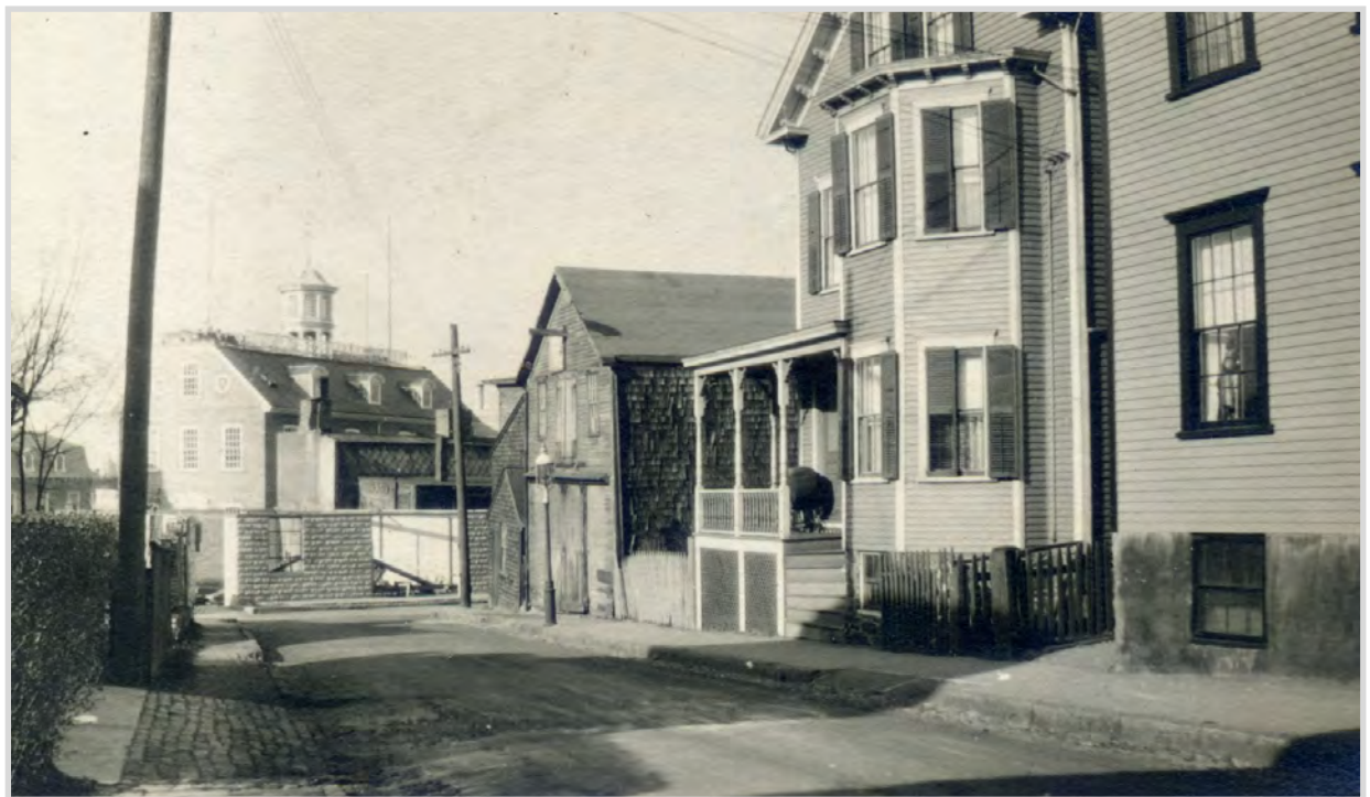
Above: Construction of gas station showing old livery building on Barney Street, 1920s.
